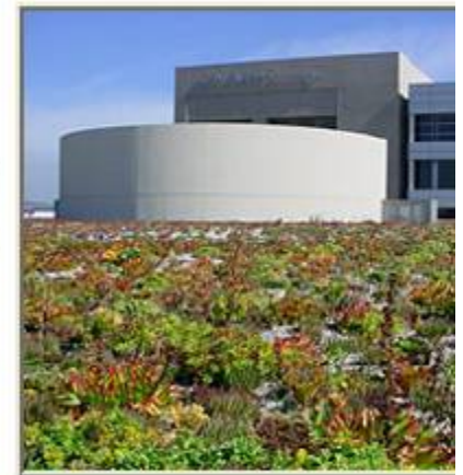
A green roof sits atop Ford's Premier Headquarters in Irvine, CA Photo Credit: Roofscapes Inc.
